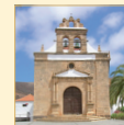
Church of Our Lady of the Rock, Vega del Río Palmas (Fuerteventura)
