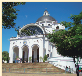
In 1840 began the construction of the grandiose Shrine with five naves. Every year, on the occasion of the Feast of the Immaculate Conception, which is also a national feast, more than 100,000 people come together at the Shrine, many of them cover, on their knees, the 1.5 km that separate the holy place from the town square.
