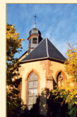
In the course of the centuries the first Chapel was destroyed due to the Thirty Years War. It was then rebuilt. Currently it is supported by the Redemptorist fathers
